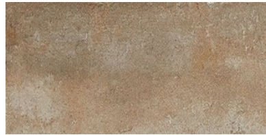
Brickwork – Patio BW03
